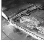
If using the frame on the outside of the duct, a continuous liquid tight weld is required. Care should be taken to not warp the frame when welding.
