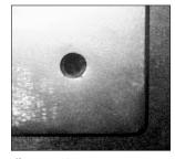
4b. CENTERED If you can not see the wall of the duct through any of the corner holes. then it is centered.
