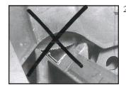
2. Never cut WDCI angle with legs up as chips may fall into the mastic.
